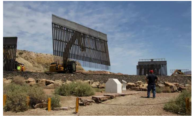
U.S.-Mexico border wall construction near Ciudad Juarez in May 2019.
