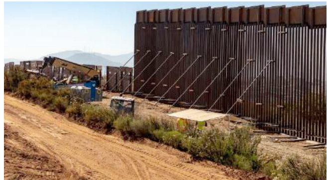
CBP announces 65 miles of new border wall construction in Rio Grande Valley Sector.
