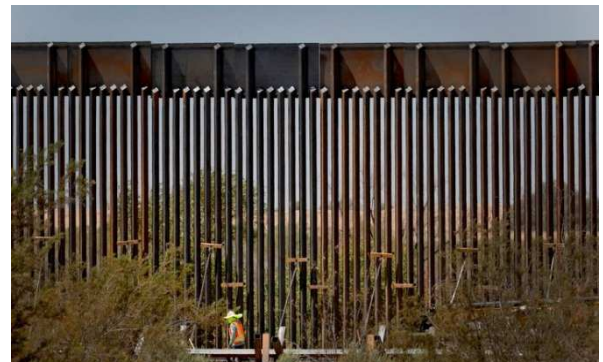
A government contractor walks beside a completed section of Pentagon-funded border wall along the Colorado River this month in Yuma, Ariz.
